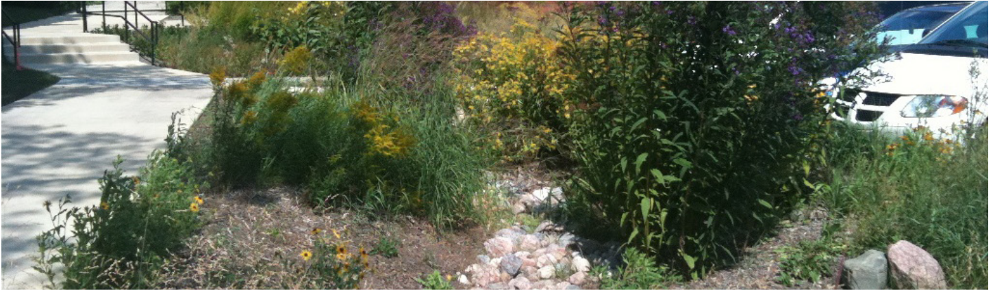
Bioretention area integrated into a parking lot at the University of Wisconsin.
