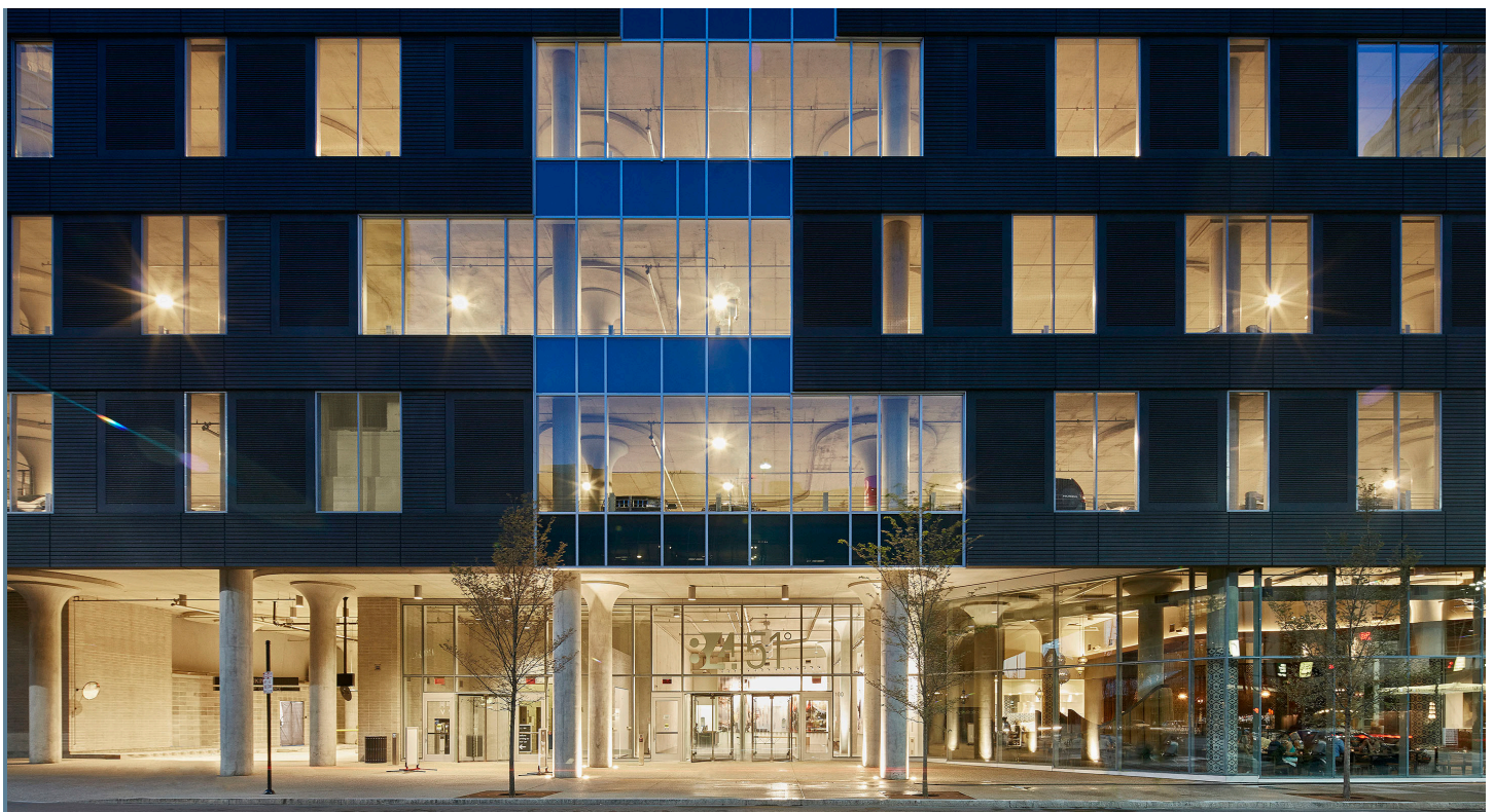
Three floors of discreet parking nestled between the ground floor and the upper office floors, Cincinnati Source: Garrett Rowland, Gensler
